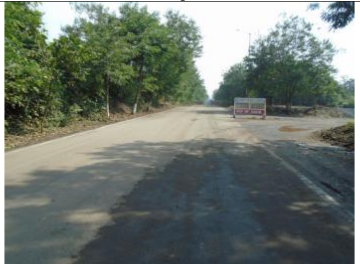
Way to Admin Building
