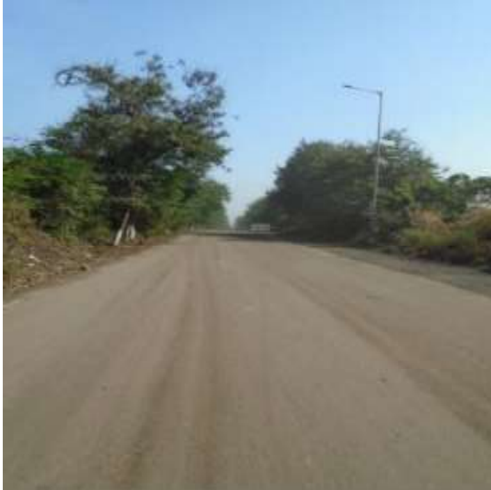
Way to Power Plant
