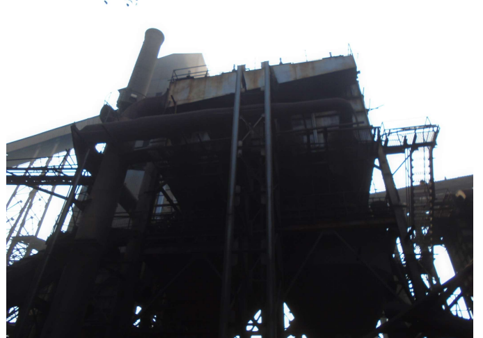
(fig. 8: DRI New Bagfilters - Cap:85,000m3/hr)
