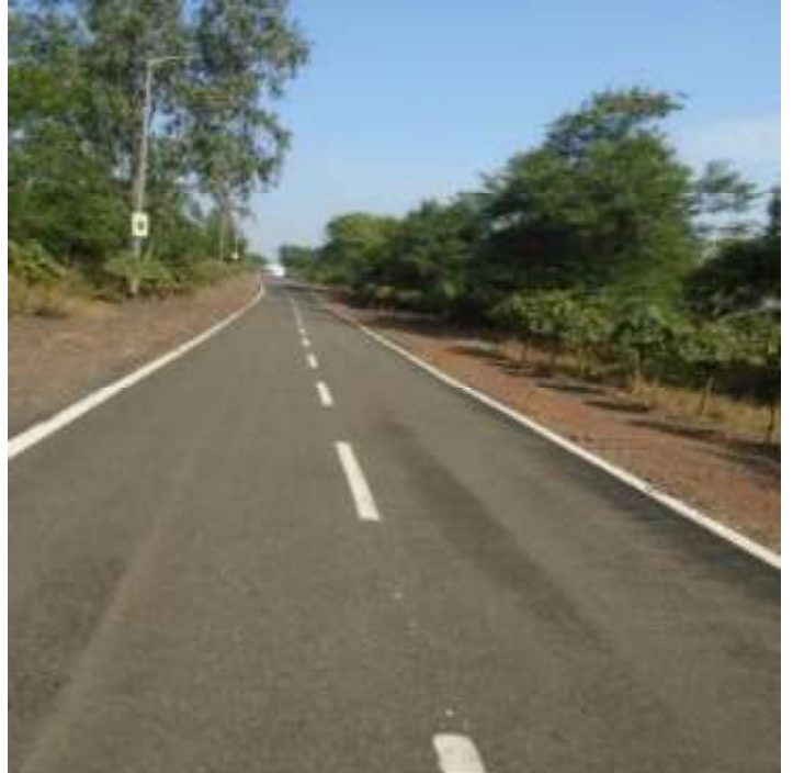
Guest House to Main Gate
